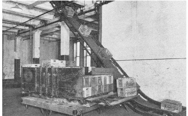
*Cases of empty bottles are unloaded from the body and placed on an escalator to the second floor of the factory where the cases are filled with full bottles.*
