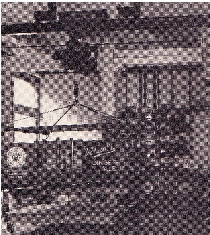
*The empty body is loaded from a gravity roller type of conveyor*
